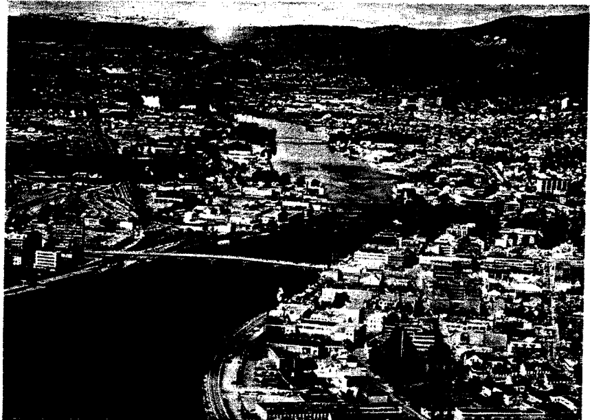
Fig. 6. The Drammen River, Norway, developed for hydro-power production with environmental considerations.
