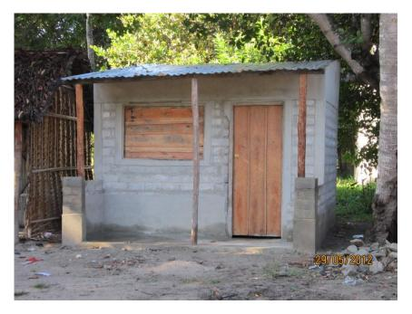
Photo 7: A local shop made from LCC bricks
