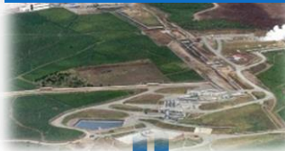
Kamojang 235 MW West Java
