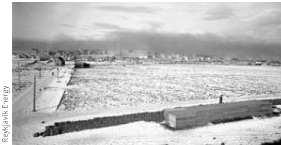
A black cloud of smoke over Reykjavik in 1940, due to heating with coal
