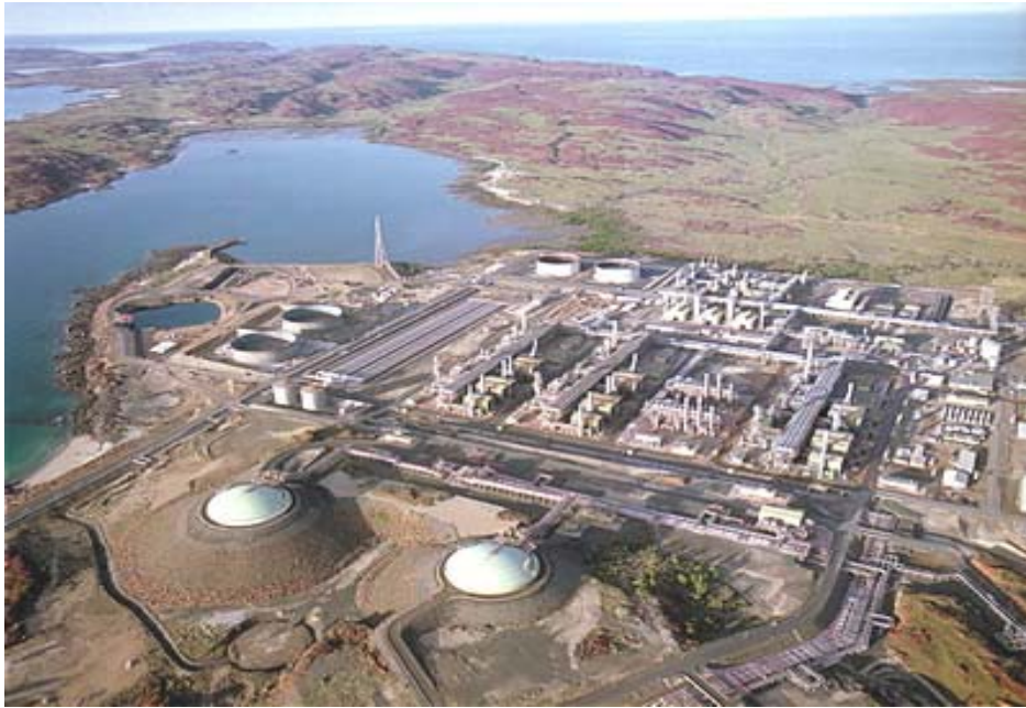
Figure 3.13: LNG plant in Western Australia
