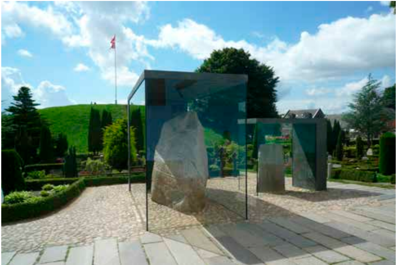
FIGURE 4.2 Protective coverings for the two rune stones at Jelling were erected in 2011 to ensure a controlled environment and to prevent damage to the monuments. ©Anne Pedersen.
