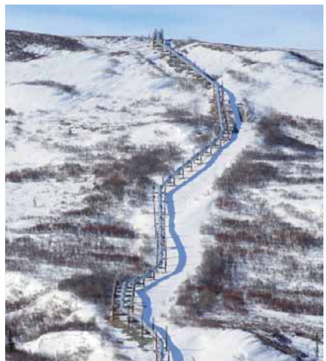
The Trans-Alaskan Pipeline.
