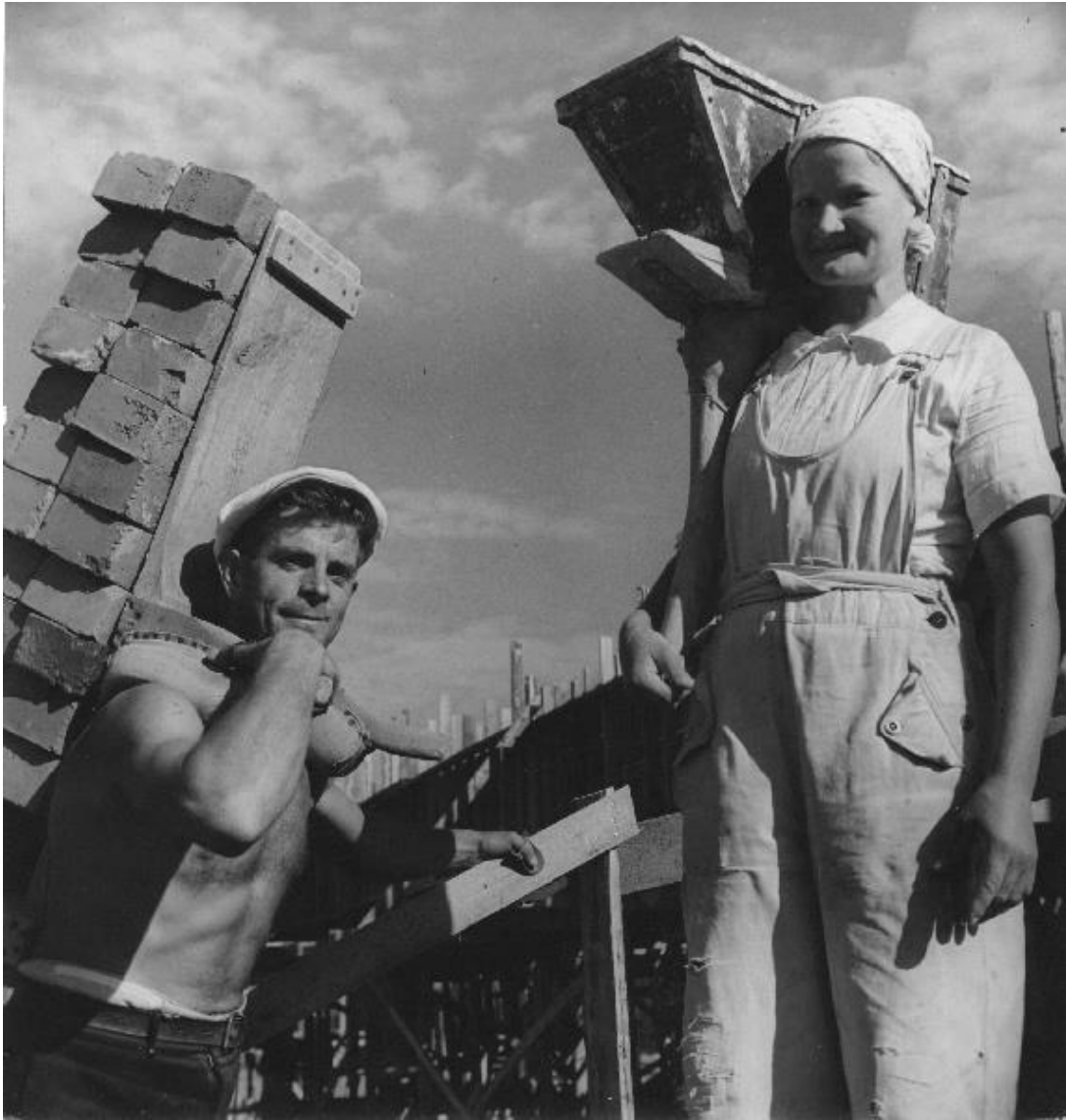
Builders at a construction site in Helsinki during the World War II. The Labour Archives.
